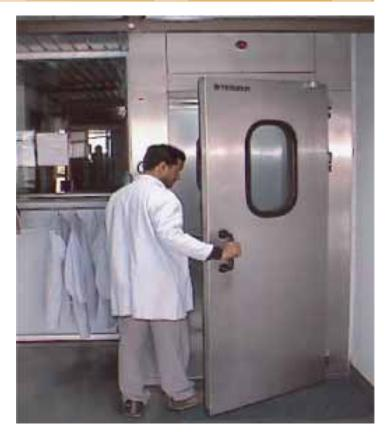
Second entry level to the NPF where every individual is air showered and vacuumed to remove any particulate contamination.
