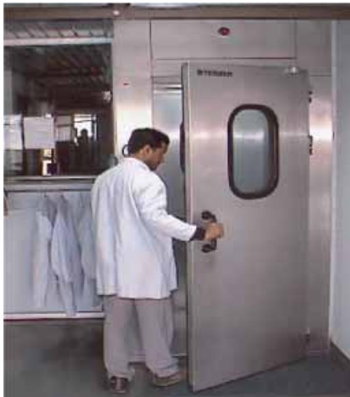
Second entry level to the NPF where every individual is air showered and vacuumed to remove any particulate contamination.
